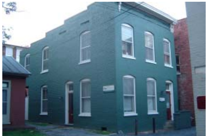
VCC's office at 17 Barristers Row
