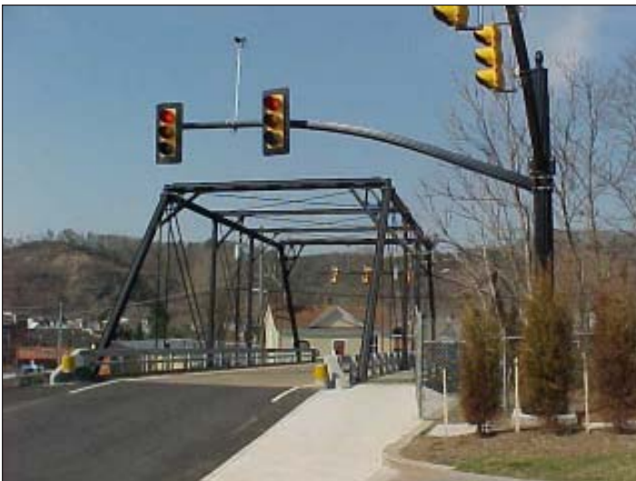
Hawthorne Street Railroad Crossing, Covington
