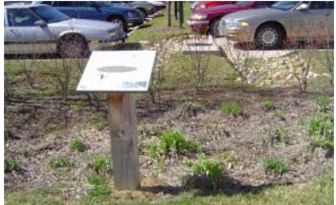
This rain garden absorbs and filters the runoff from the adjoining parking lot.
